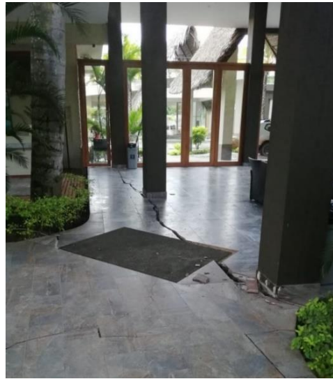
Fig. 13. Lateral spreading with cracks at the “El Sauce” Resort in Tarapoto
