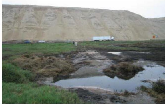
Fig. 10. 400-m slope failure along the Pan-American Highway
