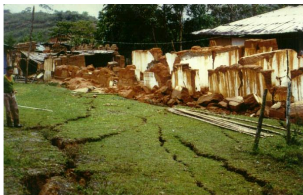
Fig. 5. Damage to mudwall houses and ground cracking due to lateral spreading in Azunge.
