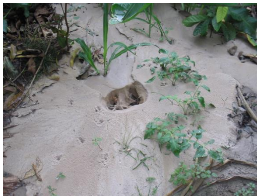
Fig. 9. Sand boils, city of Moyobamba
