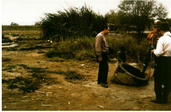
Fig. 3. Damage to sewer inlets due to liquefaction
