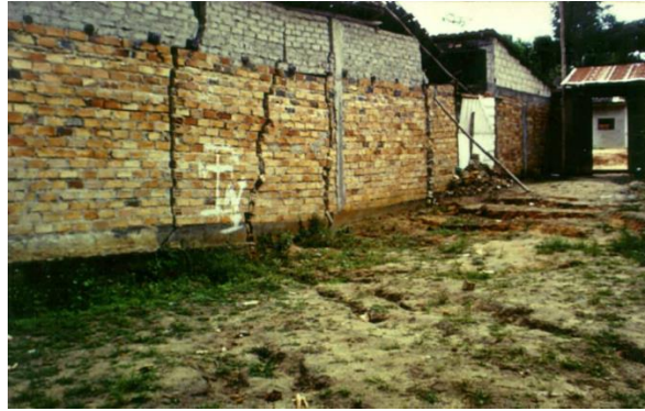
Fig. 6. Ground cracking due to liquefaction going through a brick wall in Shango
