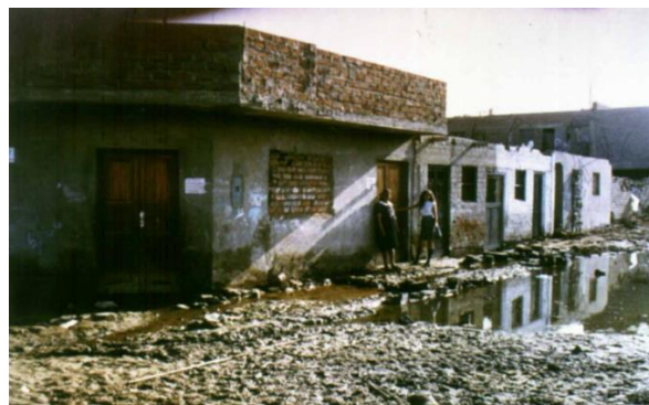
Fig. 2. Flooding of area in southeast Chimbote due to settlement and soil compaction.
