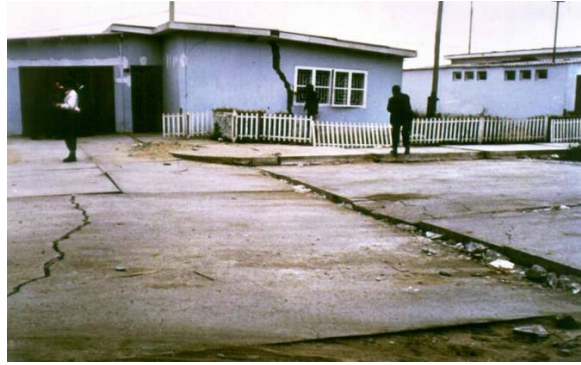
Fig. 1. Concrete-block house affected by differential compaction and lateral spreading due to the liquefaction of beach sand.
